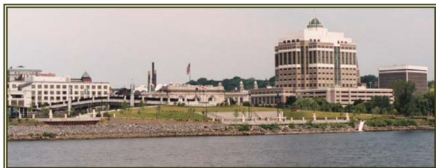
Recently completed pedestrian bridge and amphitheater at the Corning Preserve – just south of the proposed boathouse site.
