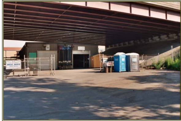
Existing ARC boat storage facility underneath Interstate 787.
